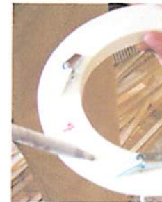
Step #5 Apply appropriate adhesive (see chart) to the bottom of the base ring as shown. Install the base ring by inserting the toggle bolts into the wall and tighten in place. Note: Remember when attaching the base ring to the wall, ensure it is lined up with the base ring circle that was drawn earlier.
