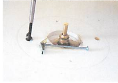
Step #3 After using the base ring to mark the location for the mounting bolts, drill the four holes using a 5/8" drill bit. Note: This is for hollow wall applications using toggle bolts. If installing the base ring to a wooden stud, recommend using 3" screws. Never use plastic mollys anchors for installation purposes.
