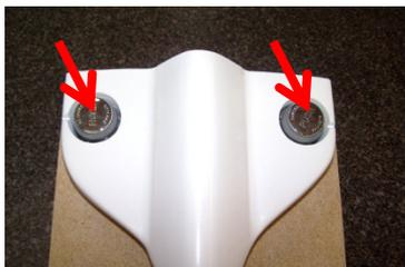
12. Make sure the faucet handles are still centered in each hole. Push down on each handle to ensure they move freely up and down. If not, you need to loosen the pipe fittings to readjust.
