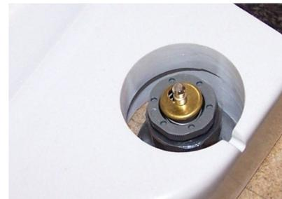
8. Install the top portion of the handle assembly into the receiver as seen in this photo. **Make sure all fittings are tighten with the proper plumbing tools and not by hand.**
