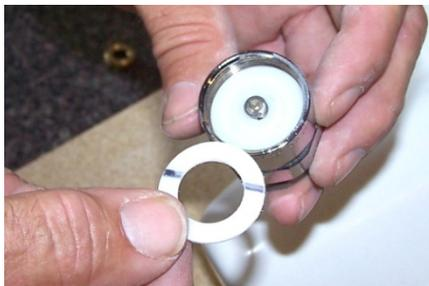
7. Before installing the top section of the faucet handle, make sure this white gasket is installed first. Please note the gasket markings indicate which side the gasket goes into the fitting.
