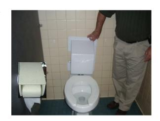
5) Level the top of the cover before attaching to the wall to ensure it is parallel to the floor.
