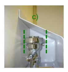
c) Depth of plumbing tree?(i.e. wall to outside of valve)
